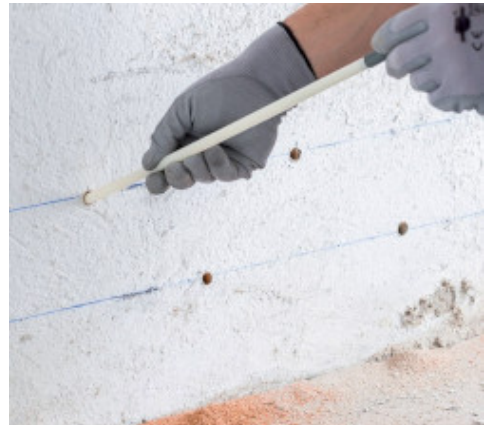
Inserting the injectors in the holes
