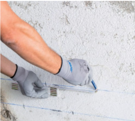
Preparing the holes
