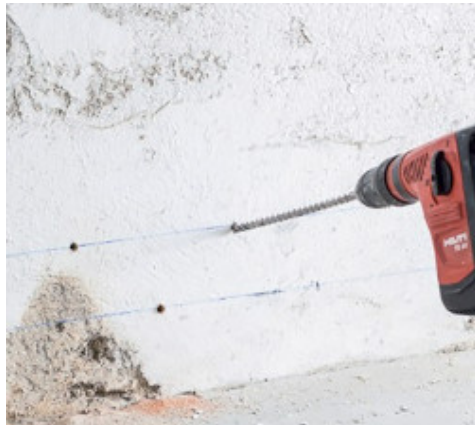
Drilling the holes
